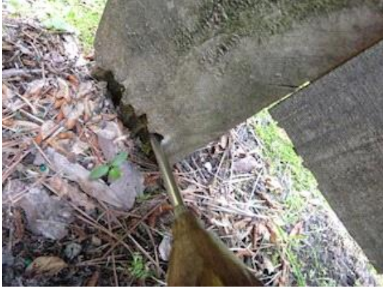
Fences / Gates - Rear: View showing water-damaged wood
