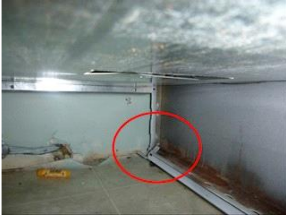
Kitchen: View of missing anti tip device located under the kitchen stove
