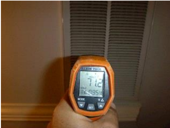
Cooling: View of return air temperature using a digital thermometer in the cooling mode
