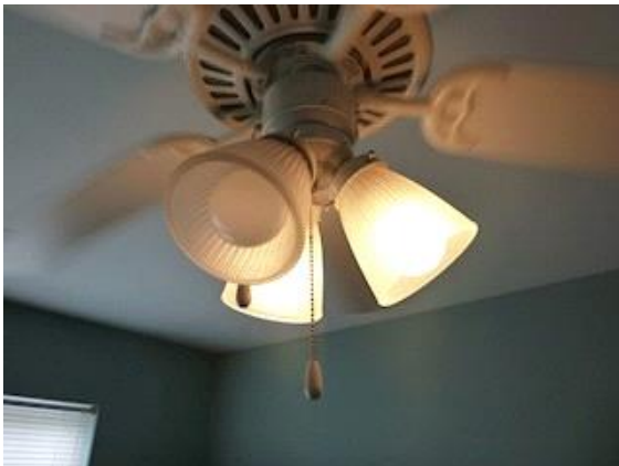
Bedroom #2 - 2nd Floor - Left: View showing defective ceiling fan light
