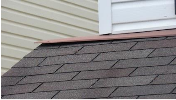
Flashing/Valleys: View showing lifted flashing
