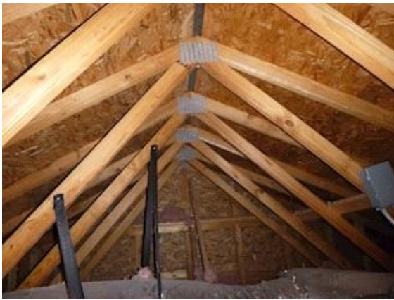
Attic Framing/Sheathing: Views of attic framing and sheathing
