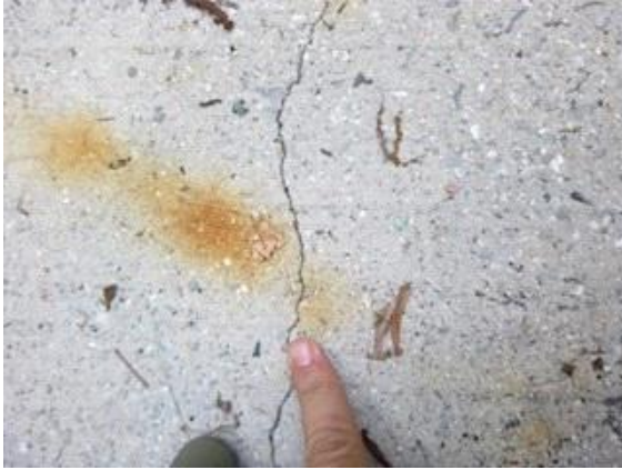
Patio - Rear: View of minor cracking present in concrete patio
