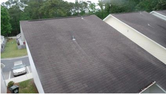
Roofing: Overall views of asphalt roof shingles
