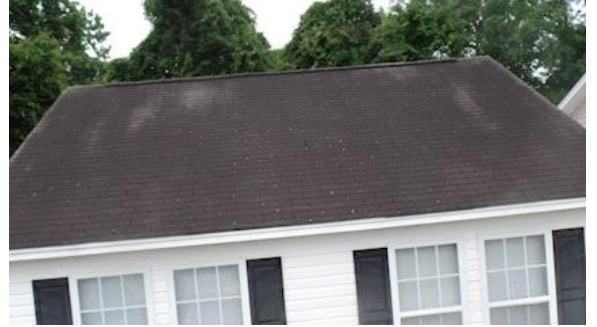
Roofing: Overall views of asphalt roof shingles
