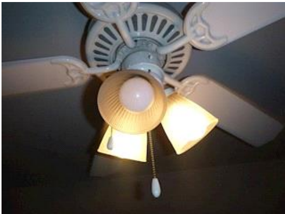
Bedroom #3 - 2nd Floor - Right: View showing defective ceiling fan light
