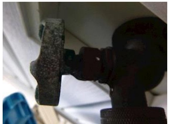
Exterior Surface: View showing leaking faucet
