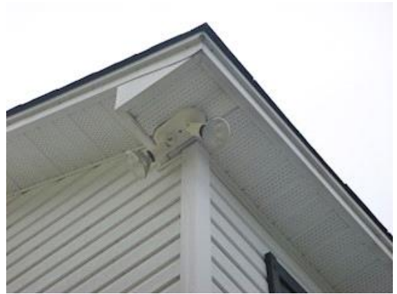
Exterior Surface: View showing defective spotlights
