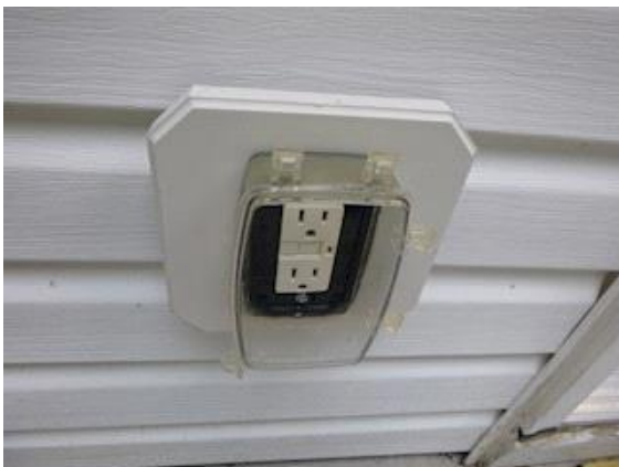
Exterior Surface: View showing missing receptacle cover
