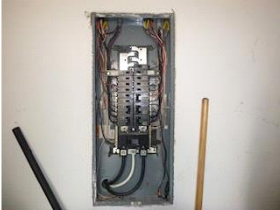
Electrical: View of main electric panel and circuit breaker located in the storage room
