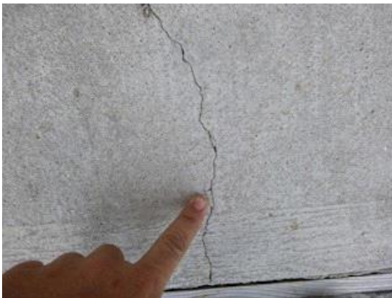
Porches / Stoops: View of minor crack on front porch
