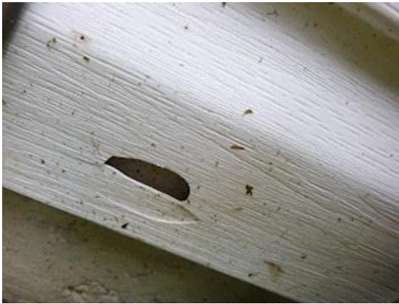
Exterior Surface: View showing cracked siding
