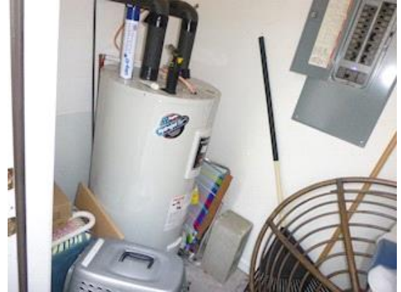
Water Heater: Overall view of water heater
