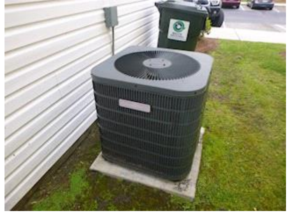
Cooling: View of HVAC condenser located on the left side of the house
