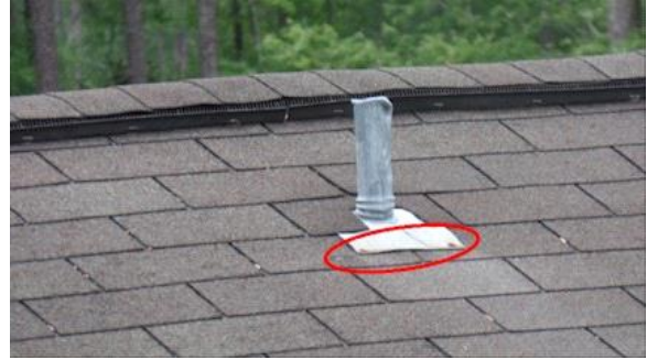
Flashing/Valleys: View of exposed nail heads at the base of vent pipe flashing
