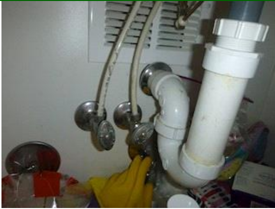
Plumbing: View of plumbing pipes below sinks
