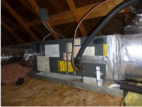
Cooling: View of air handler located in the attic area
