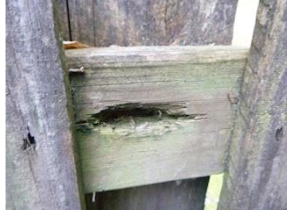
Fences / Gates - Rear: View showing damage due to insects
