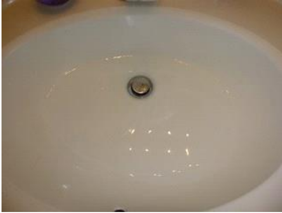
Bathroom #2 - 2nd Floor: View showing slow draining sink
