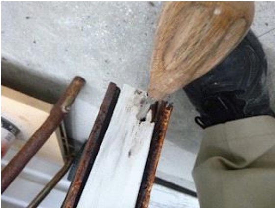
Exterior Doors: View showing water-damaged door core
