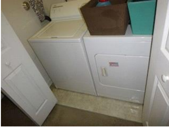
Laundry Facilities: View showing missing drain pan under washing machine
